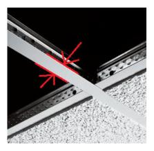
Two "L" shaped side rails are provided. NOTE: these are to be installed first. The "L" side rails sit atop the 4ft sides of the grid and are held in place at the ends by the "Lift" Rails. After "L" side rails are installed, proceed to step 3. of the installation found on page 2.
