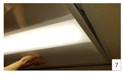
6<sup>™</sup> closest you to clear the T-Bar face. Raise the non-hinge side above the T-Bar and slowly pull back until you feel the hinge bolts drop into the locking slot (8). The KuDo 6<sup>™</sup> may now be allowed to rest on the T-Bar (9).
