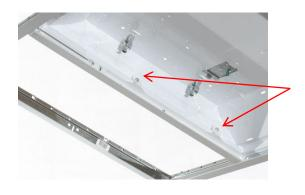
Check to make sure the old fixture is connected to the building structure with No. 12 hanger wire as per code. Permanently fasten the "LIFT RAILS" by drilling a self-tapping screw through both screw tabs into the old troffer housing as shown left. Do this for both Left and Right "LIFT RAILS".
