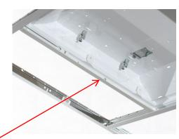
Fasten LIFT RAIL to the T-Bar by drilling a self-tapping screw through one of the pilot holes provided in the middle of the LIFT RAIL. Repeat Step 4. for the second LIFT RAIL on the opposite side.
