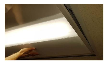
drop into the "Drop Slot". The KuDo 6T™ may now be allowed to rest on the T-Bar (9).
