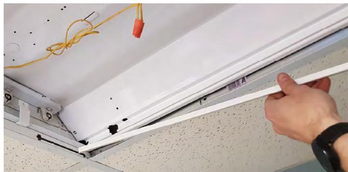
The K6L-SR has fingers on the ends that fit into the LIFT RAILS and slide into place as seen above.
