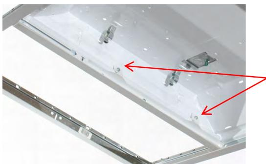
Check to make sure the old fixture is connected to the building structure with No. 12 hanger wire as per code. Permanently fasten the “LIFT RAILS” by drilling a self-tapping screw through screw tabs into the old troffer housing as shown left. Do this for both Left and Right “LIFT RAILS”.
