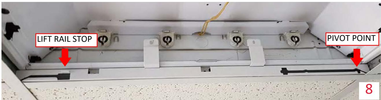
**Step 8.** Remove protective plastic from lens and dispose. If you notice any debris on the lens, remove the lens and clean the debris. Replace lens.
