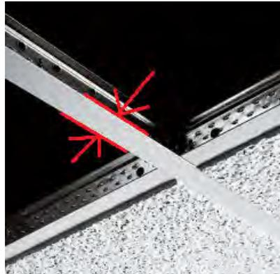
Two "L" shaped side rails are provided. NOTE these are to be installed first. The "L" side rails sit atop both sides of the grid and are held in place at the ends by the Lift Rails. After "L" side rails are installed, proceed to step 3. of the installation found on page 2.
