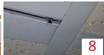
**Step 8.** Remove protective plastic from lens and dispose. If you notice any debris on the lens, remove the lens and clean the debris. Replace lens.
