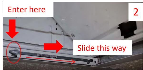
**Step 5.** (1) Lift the KuDo 6™/KuDo 6L™ fixture body so that the back is facing towards you with hinge bolts at top left and top right corners. Angle the fixture body so that the top left hinge bolt HEAD enters the LIFT RAIL slot (2). After entry, slide partially towards the end of the slot (3). NOTE: The fixture body must be held close to parallel with the ceiling and angled slightly in order to allow the top right hinge bolt HEAD to enter the opposite LIFT RAIL in the same fashion (4) (5).
