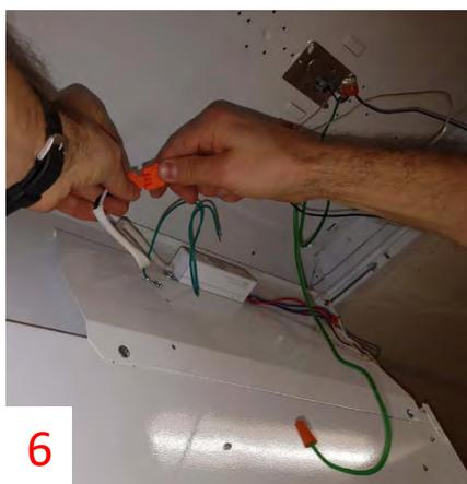
**Step 6.** After the top left and top right hinge bolt HEADS have been installed into the LIFT RAIL slots, the fixture body may be allowed to hang for hands free splicing. Fasten the aircraft cable safety tethers provided at both ends of the KuDo 6™/KuDo 6L™ body to the old troffer housing prior to splicing. Proceed with wire splicing with ground wires being spliced first. Use the power disconnect provided.
